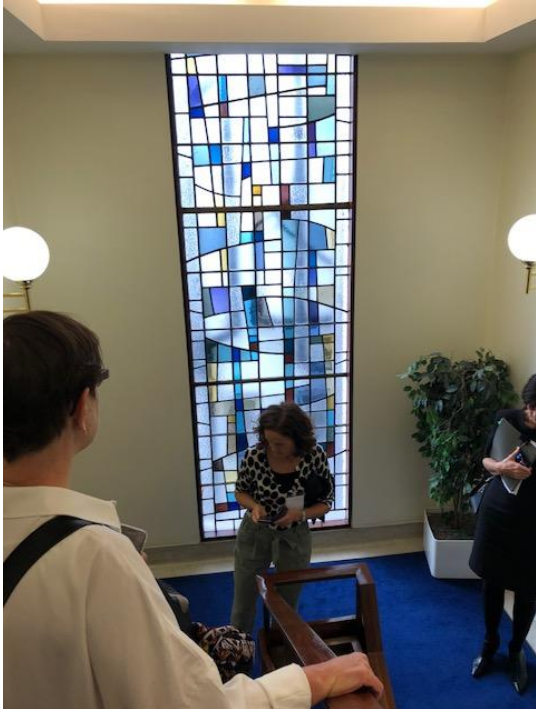
All original stained glass to Building B still exists in the main stairwell extending throughout the building
