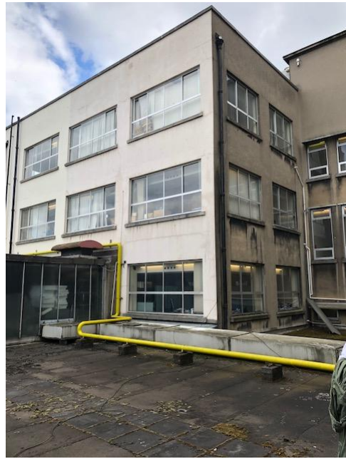
Rear of Building A onto Dawson Lane. Original Openings still intact along the rear elevation
