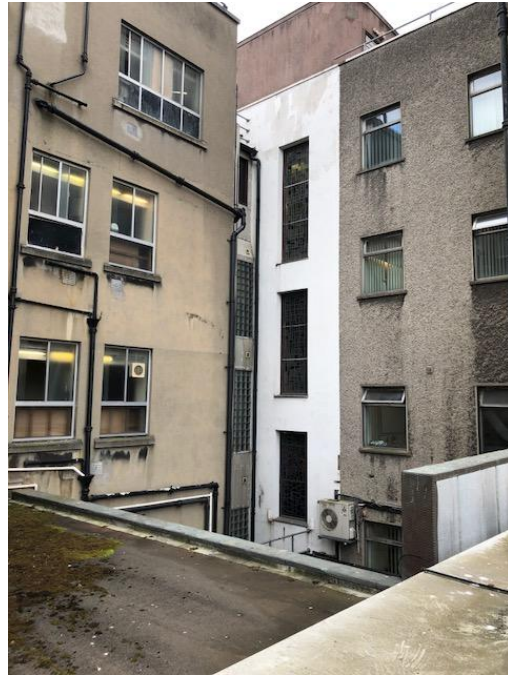
The rear of Building B showing the original stained glass windows and the glass block link element. (where the chute to the post room is located)
